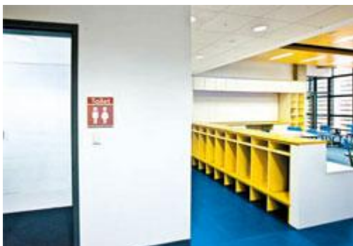
A washroom and lockers attached to an elementary classroom. Behind lockers is a kitchen sink installed.
