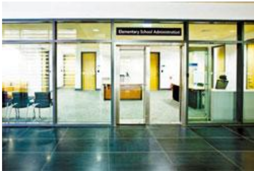
Administration office finished with solid glass walls is seen from outside.
